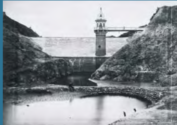
► A lone man sits on the Baker's Hill gold mining weir, which had supplied water to a stamper battery.
