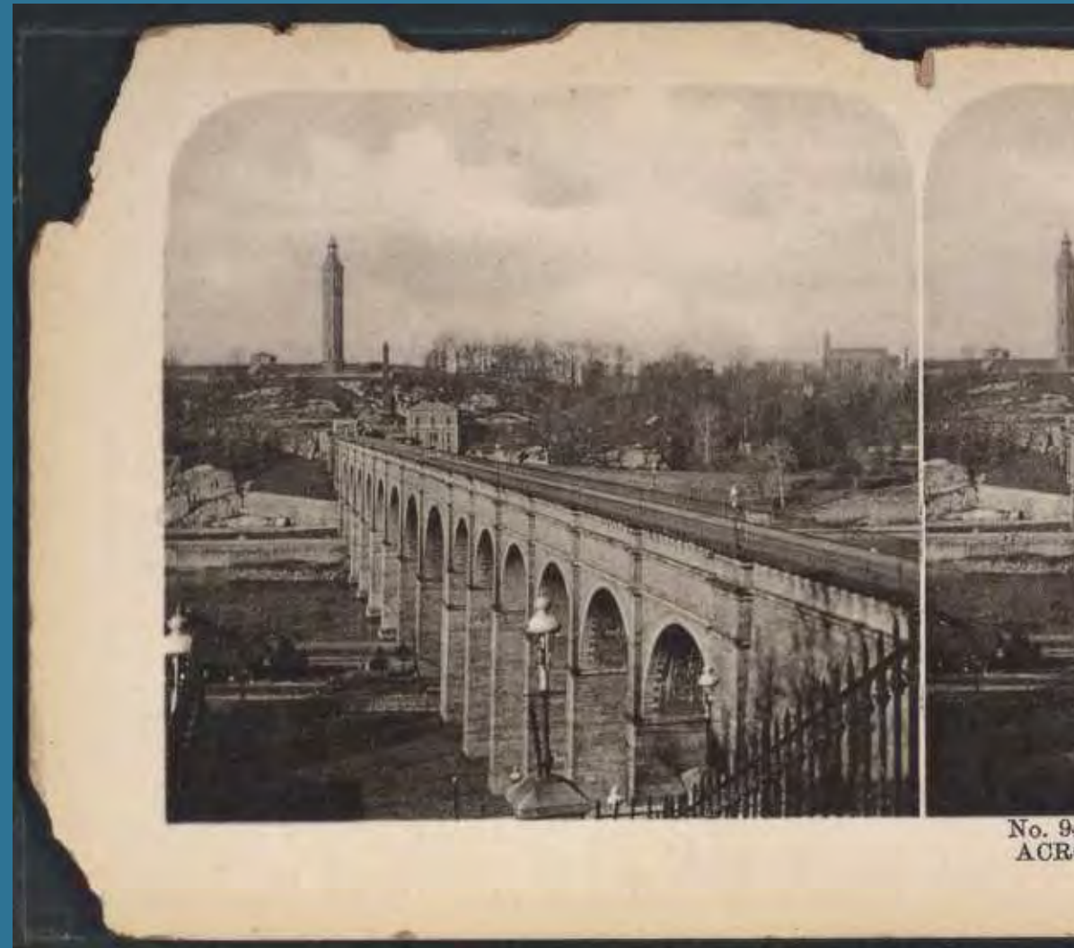
► A picture of The Old Croton Aqueduct
