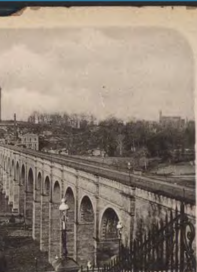
4. HIGH BRIDGE (CROTON AQUEDUCT) ACROSS HARLEM RIVER, FROM THE EAST.
